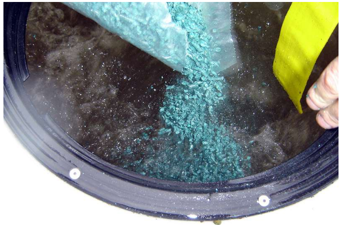
Mixing components for hydroseeding
