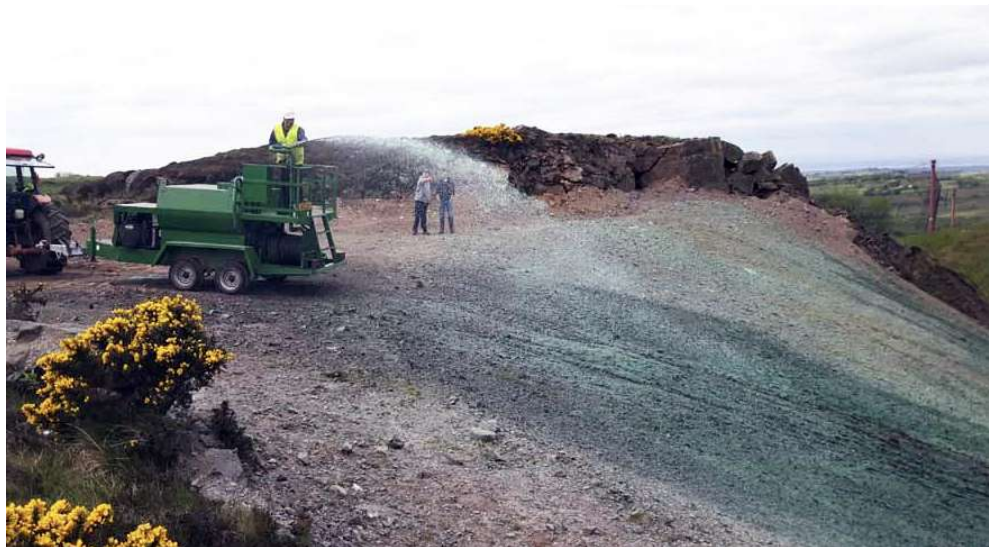
2,500 litre hydroseeder sowing steep sloping area
